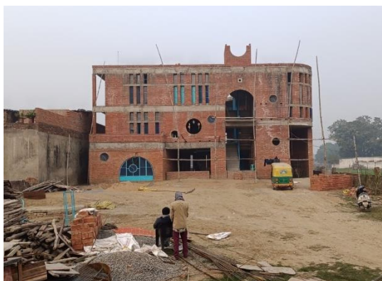
The current state of our building. Waterproofing of our roof as well as a top structure, a screen for our water tanks, was finally completed last week. Just one simple grill remains to be placed at the very top. Scaffolding has begun to be erected to allow for exterior plastering.
